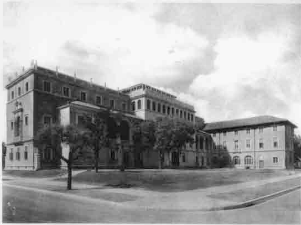
Central Library soon after opening in 1926.
